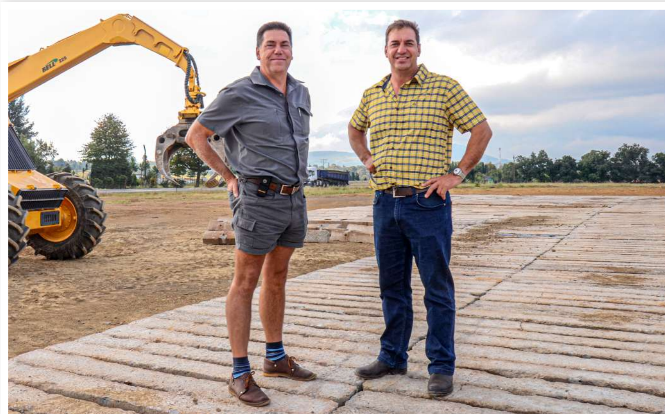
Herman (left) and Marius Brelage stand on some of the laid concrete sleepers at their developing truck stop site on the N11 outside Volksrust.
