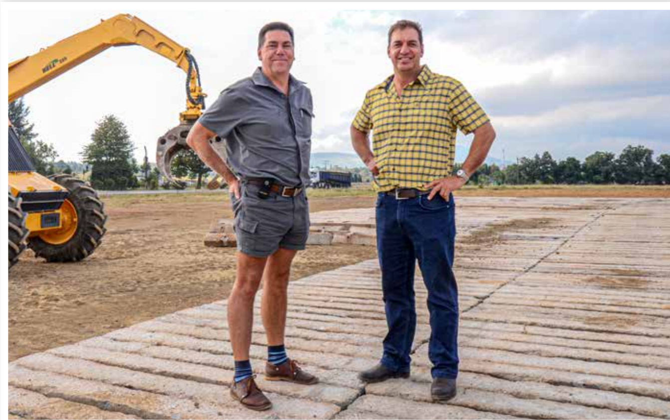
Herman (left) and Marius Brelage stand on some of the laid concrete sleepers at their developing truck stop site on the N11 outside Volksrust.
