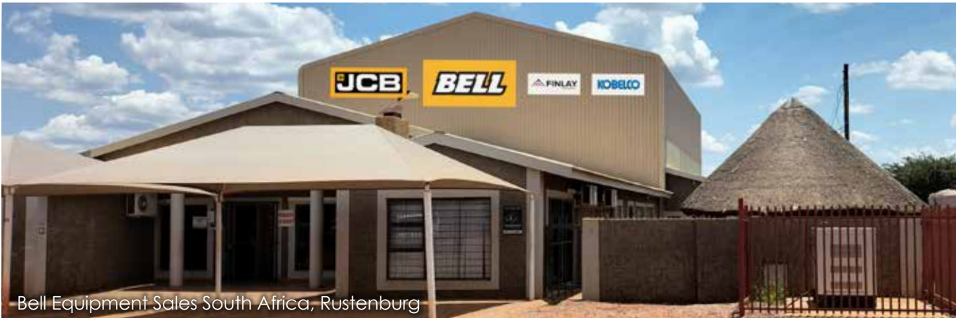
Bell Equipment Sales South Africa, Jetpark
